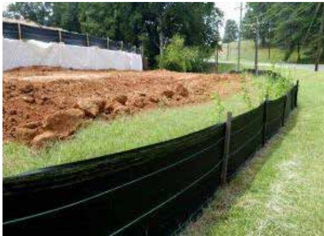
Good site management should be employed during a development's construction to retain the site's water storage and attenuation capacities and protect its SuDS, e.g. silt fences protecting infiltration components
